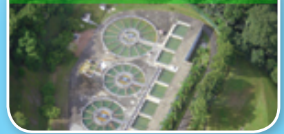
Water & Wastewater Treatment
